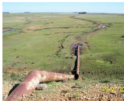
Siphon outlet and beginning of the distribution channel
