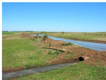
Distribution channel in operation, with lateral outlets to the fields
