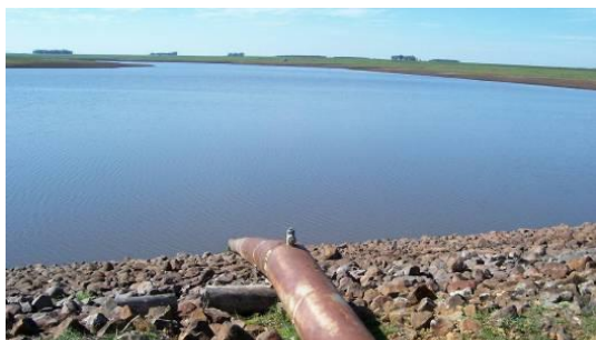
Siphon of the reservoir
